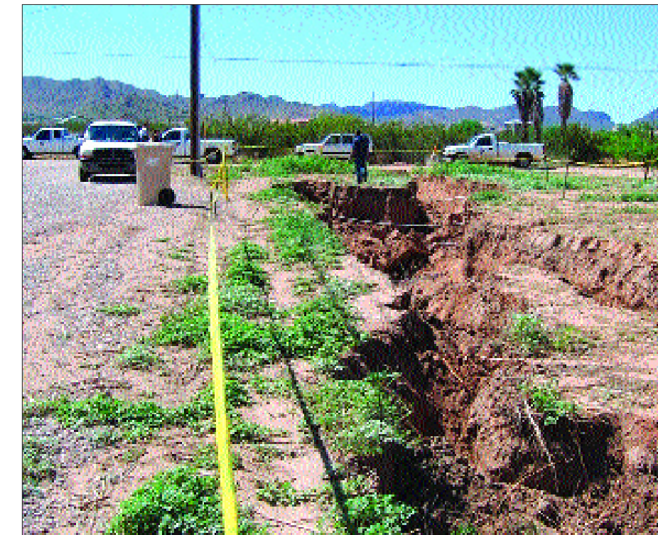
Figure 1: Earth fissure near Chandler Heights, Maricopa County, August 2005. Earth fissures range from insipid, where they are characterized by discontinuous, pock-marked ground and hairline fractures, to mature features miles in length and hundreds of feet deep, with associated gullies at the surface that are more than 10 feet wide and several tens of feet deep. (Photo by Ray Harris)
