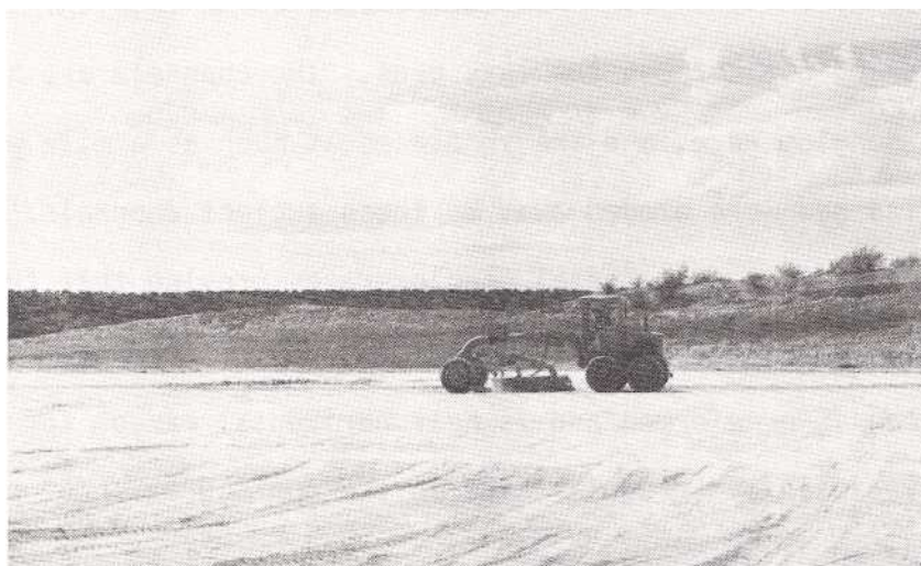
EZ 228 Pit - Cleaning Top of Beds
