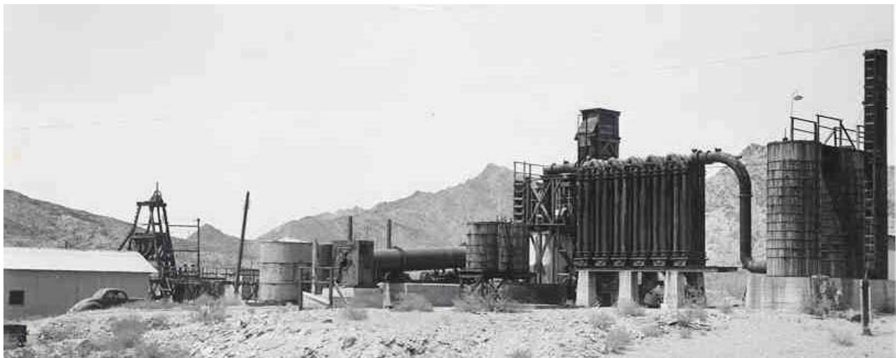
Rico Mercury Mine, circa 1930, Northern Avenue at Dreamy Draw. State Route 51 now covers the mine remains. This view is of the furnace plant and machine shop, with the headframe in the distance.
