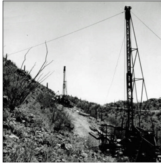
Churn drilling on Copper Girl Hill at Silver Bell, (ca. 1940s)
